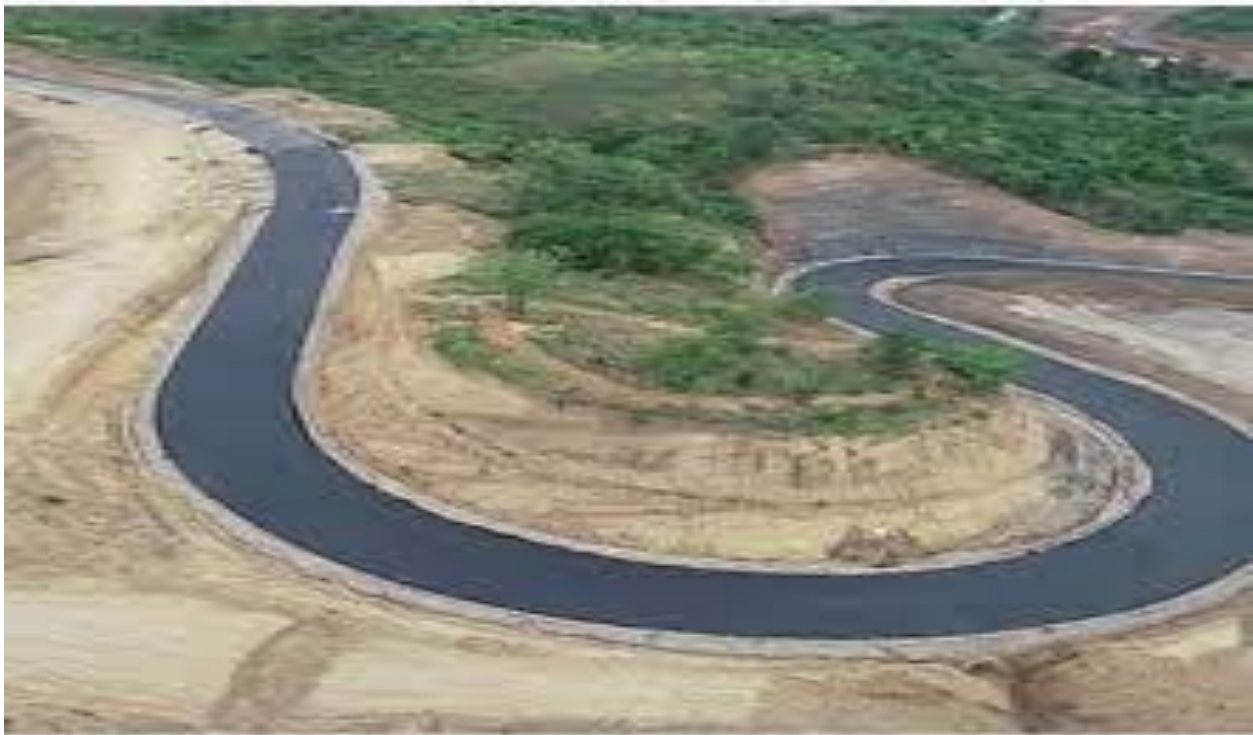
Tarmac Mbinga to Mbambabay 66km
