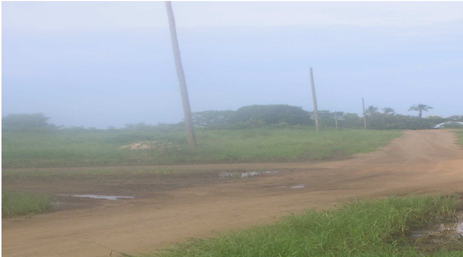
Figure 8: Power transmission line under construction in Nyasa.
